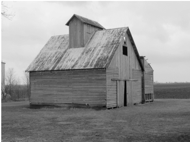
Adjacent to the crib barn at the Fritz-Heimbürger Farmstead, site 506, is a rare local example of a free-standing wood-framed corn crib.
