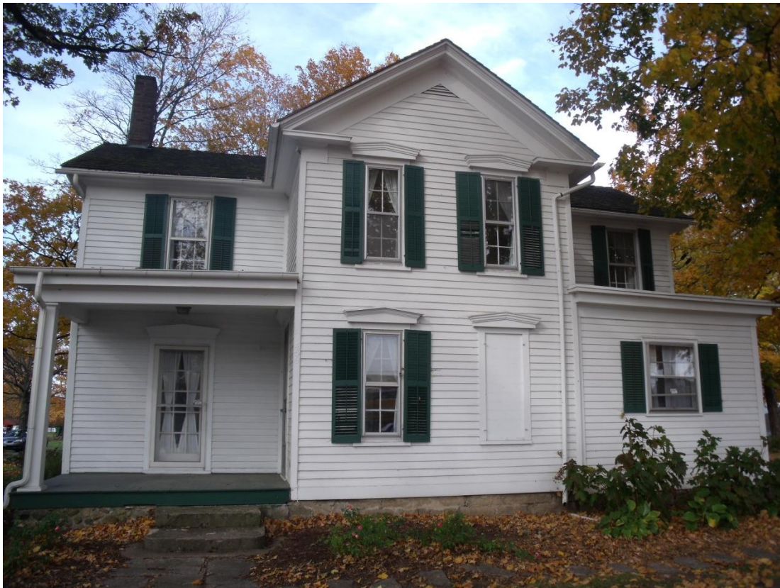
In this westward view of the farm house, gabled pediments can be seen above the windows and former doorway—a characteristic of the Greek Revival architectural style. In the 1860s, the front door was blocked off in order to create a new staircase, and the formal porch entrance was moved to the southeast of the house. The depicted entrance is not used by the public.
