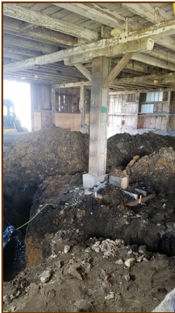
Trenches dug for water lines
